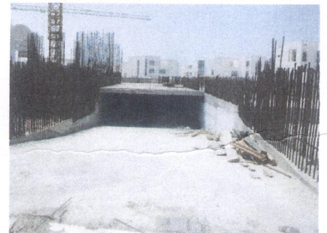
Ground Slab/Ramp To Basement
